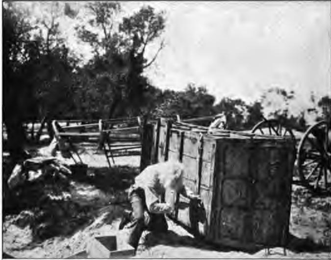
Calking the wagon box to turn it into a boat.
